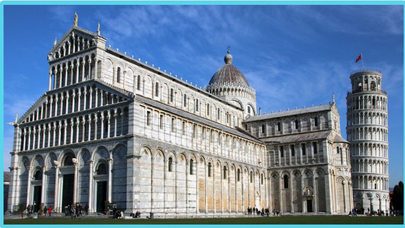
LEANING TOWER OF PISA .....
